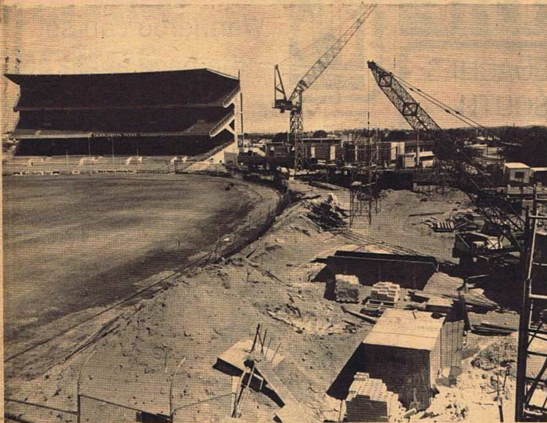
Subiaco Oval . . . the WAFL's mammoth $4 million project is well under way.
